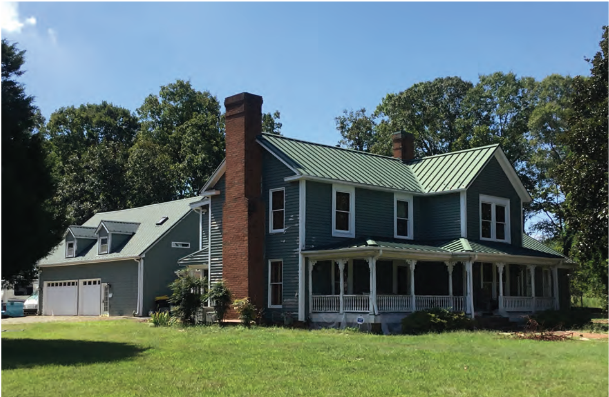
Figure 3.2. House Facade, Looking South
