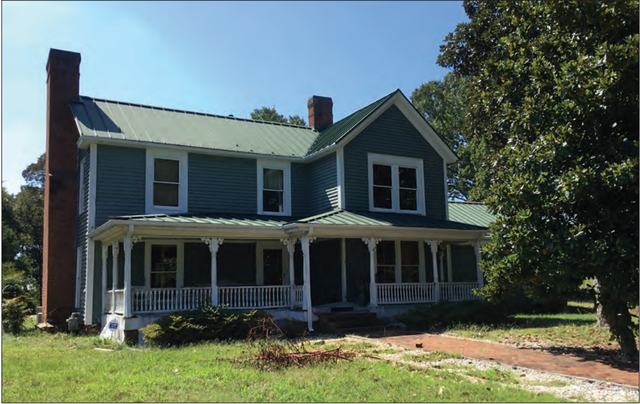
Figure 3.2. House Facade, Looking South
