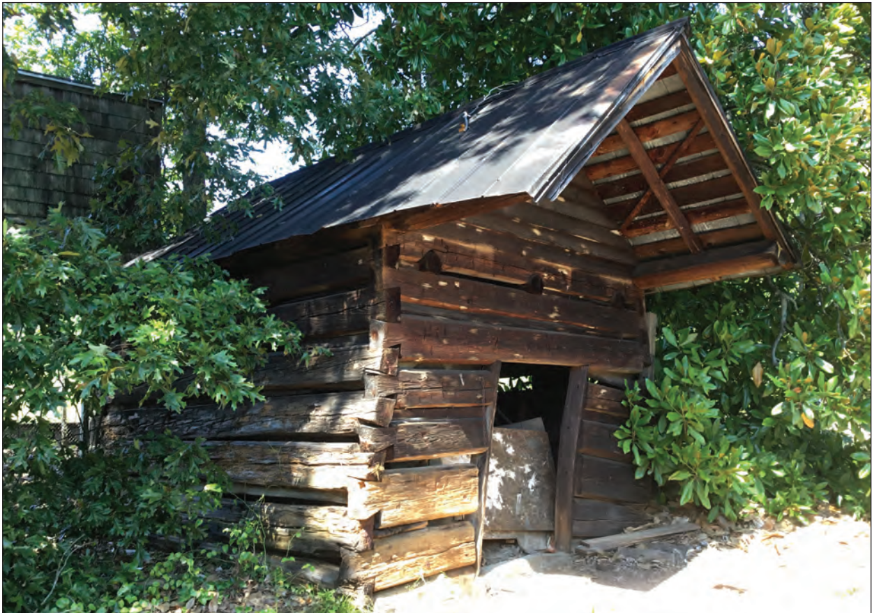
Figure 3.6. Smokehouse, Looking Northwest
