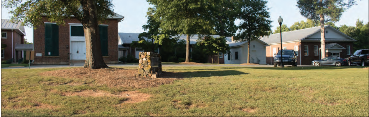
Figure 2.2. Panoramic View of Centre Presbyterian Church with 2004 Addition at Right, Looking North
