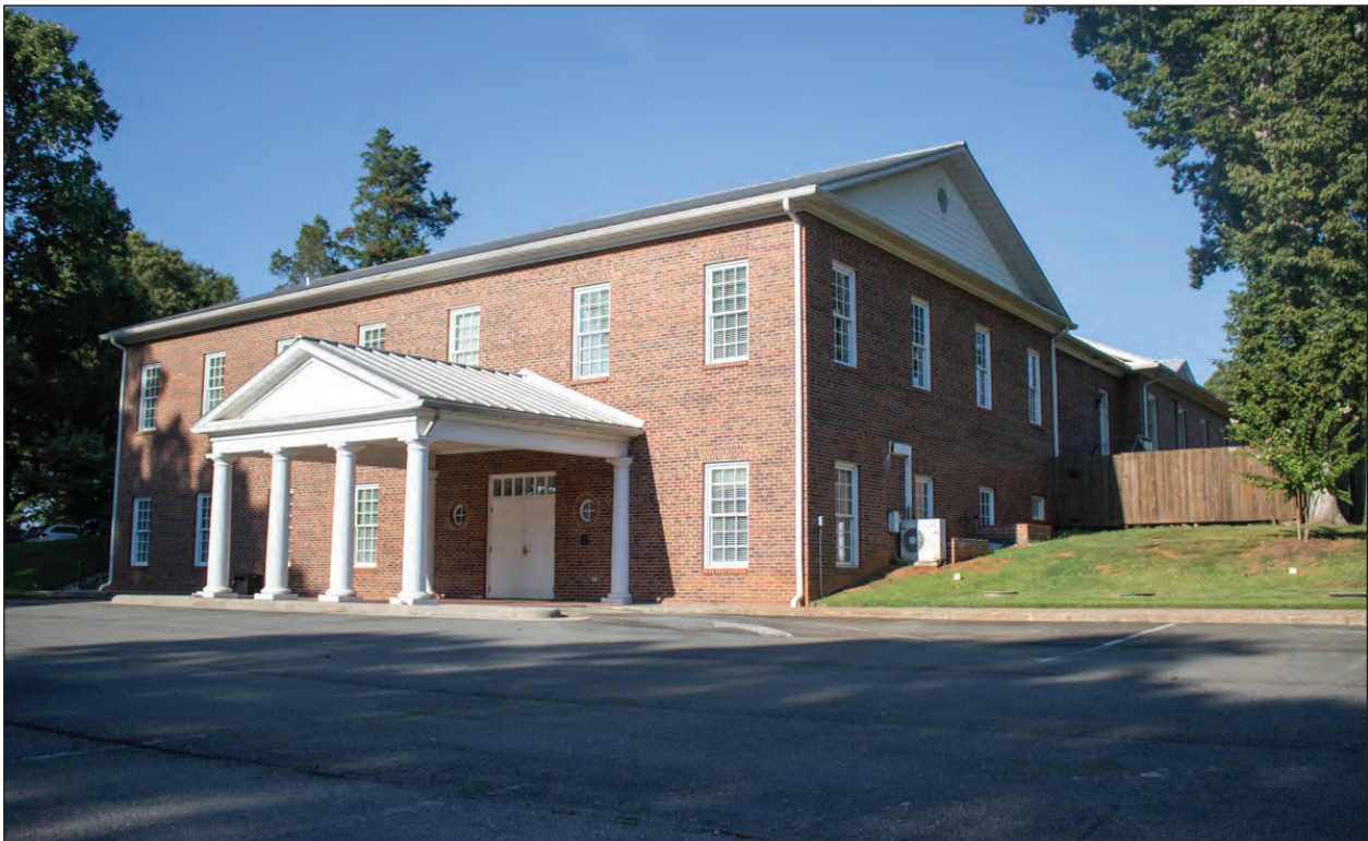
Figure 2.9. 2004 Addition, Looking Southwest
