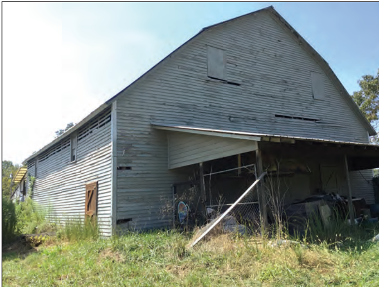
Figure 3.9. Barn, Looking East
