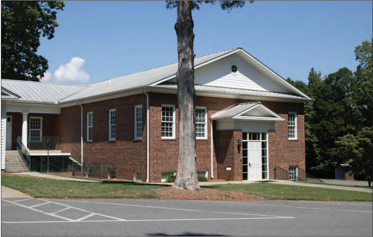
Figure 2.8. 2004 Addition, Looking Northeast
