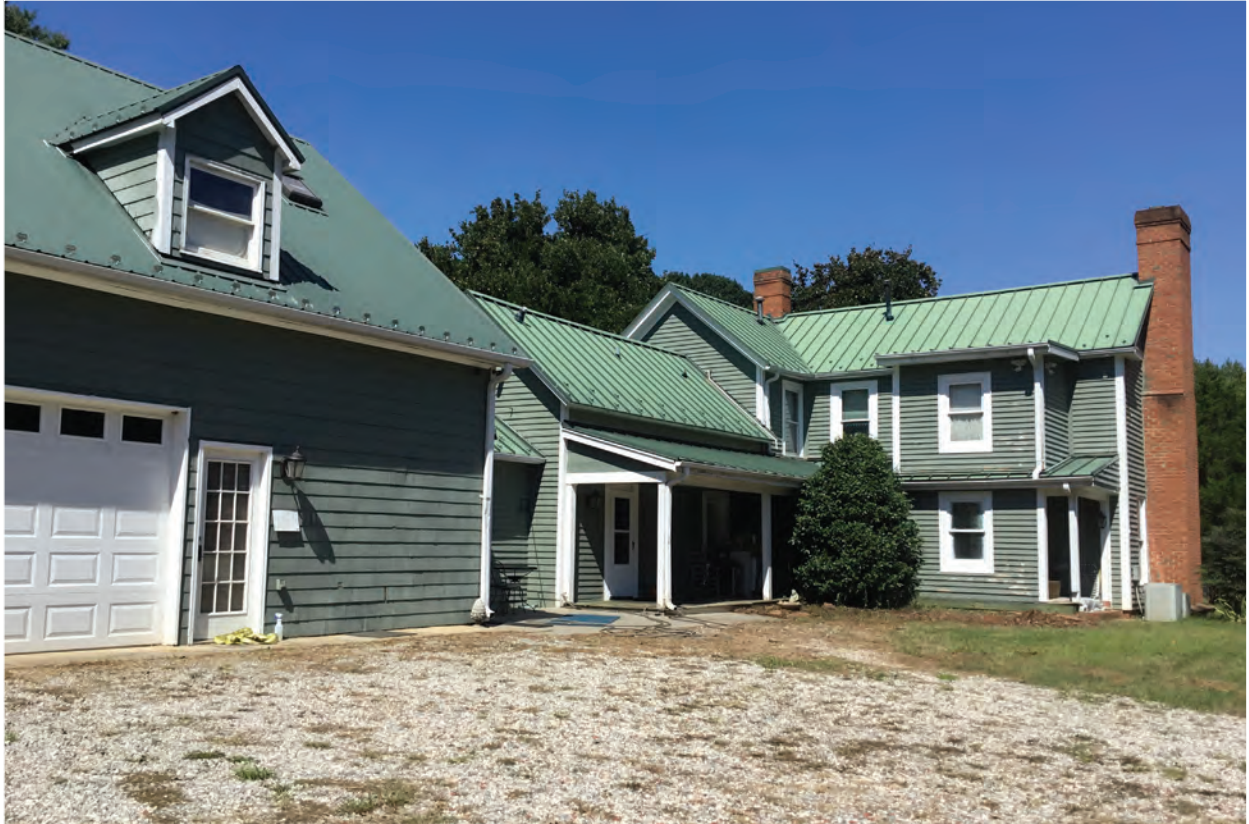
Figure 3.2. House Facade, Looking South
