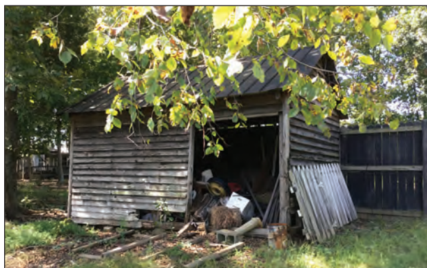
Figure 3.13. Shed Looking Southwest
