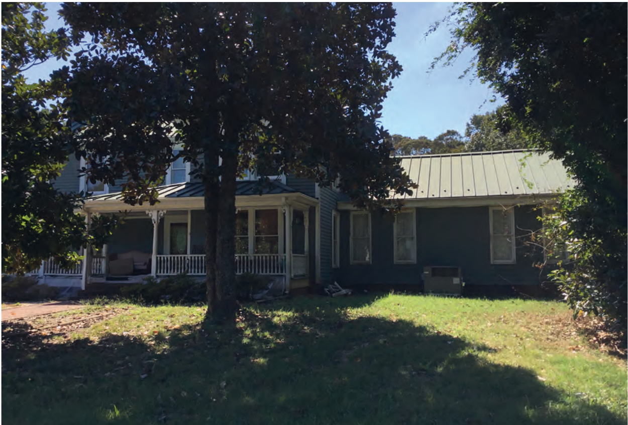
Figure 3.2. House Facade, Looking South
