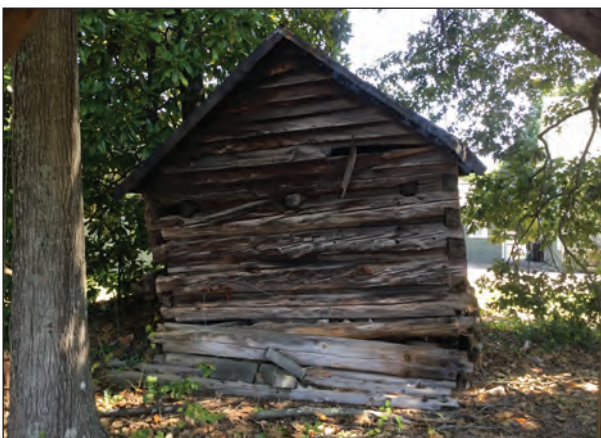
Figure 3.7. Smokehouse, Looking East
