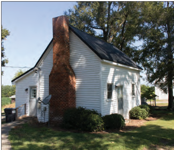
Figure 3.22 Craven-Pierce Farm, Whiskey House
